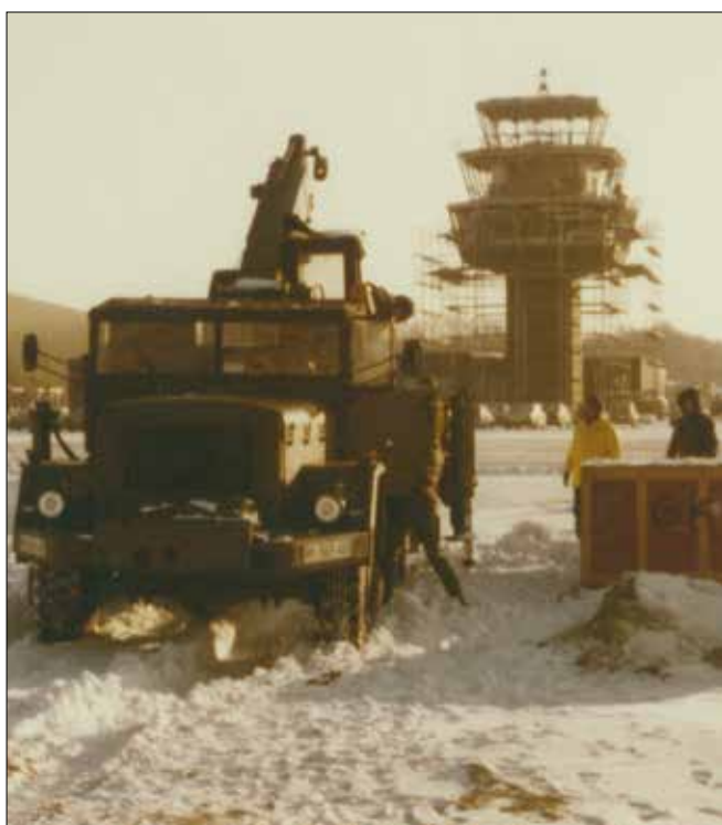
The Air Traffic Control Tower still under construction.
