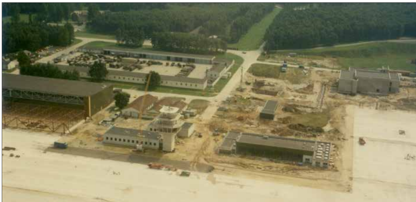
Overview of the construction site showing Hangar 2, the Air Traffic Control, Tower and the Crash and Fire Department
