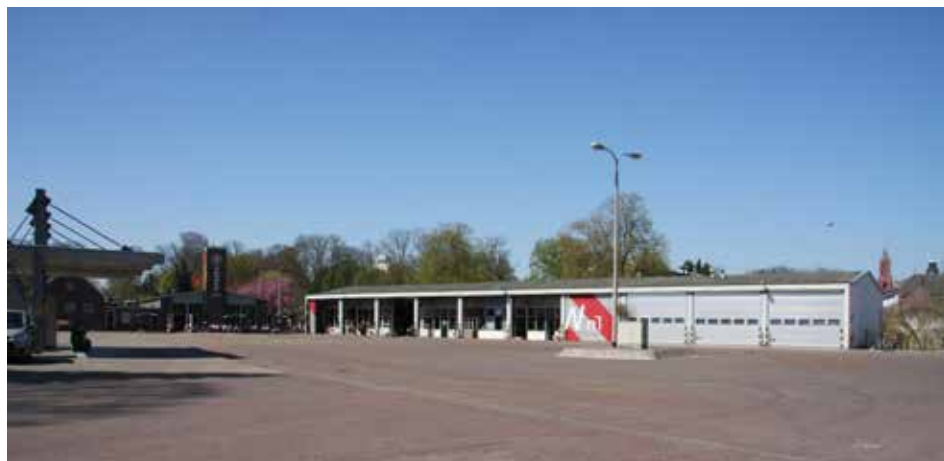
The Tapijn Casern has become a public place. The former garage building is adapted into a building for special craftsmen. It is now called "Het Werkgebouw"
