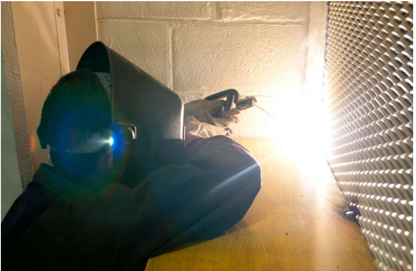
Hessian Mohammad, an Afghan National Army sergeant and welder, secures shelves in a detainee housing unit in the Afghan National Detention Facility-Parwan. Mohammad works in the ANDF-P Repairs and Utilities shop, which is responsible for facility maintenance and improvements. The shop made the transition from being U.S.-led to Afghan-led in March 2013. Photo by U.S. Army Sgt. Katie D. Summerhill, department of defence
