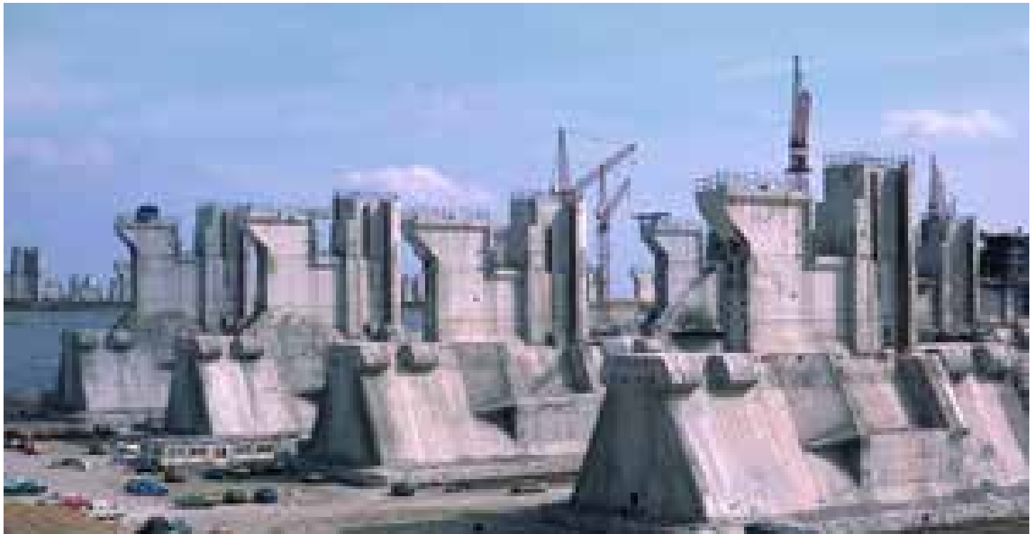
The 65 pillars of the Easter Scheldt storm surge barrier dam with 62 steel doors are each 42 metres wide, between 35 and 38.75 metres high and each weighs 18000 tonnes.
